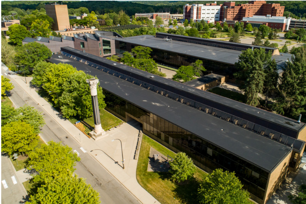
Art & Architecture Building | By Michigan Photography
